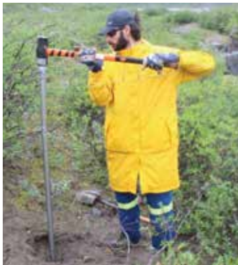
PhD candidate Milad Fakhari installing a piezometer.
